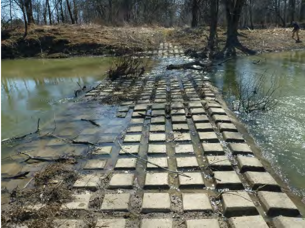
Left: Approximate location of existing low level crossing on Bear Creek. Right: Low Grade Crossing at Moore Wildlife Area, photo taken March 23, 2017
