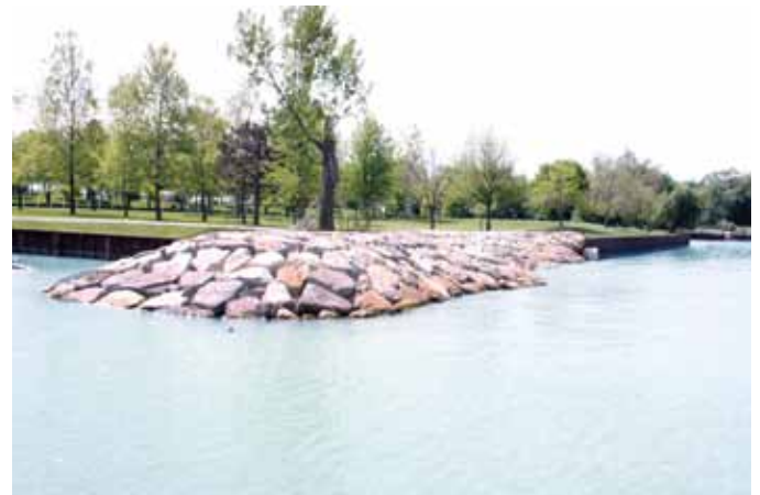
Shore protection at Cathcart Park on the St. Clair River
