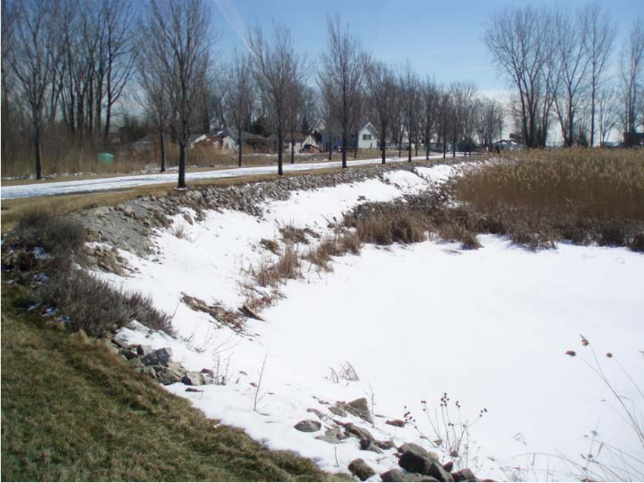
View of a dike that is also functioning as a road. The stone revetment has been placed for added protection.
