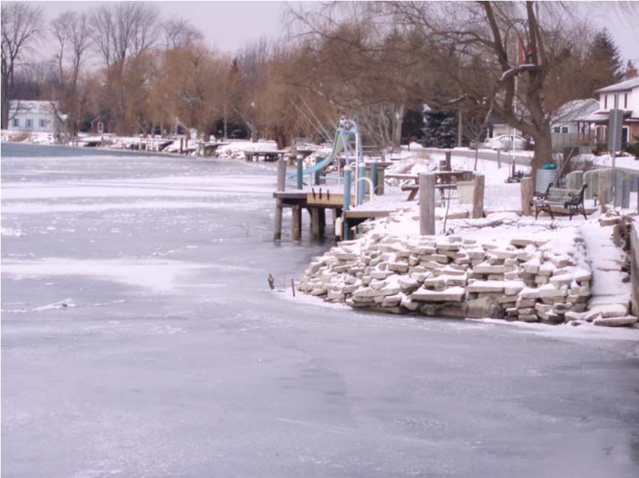
Photograph of Bluewater Line, where the road has been built on top of the dike.
